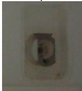
Figure 26: Internal part of vacuum port
